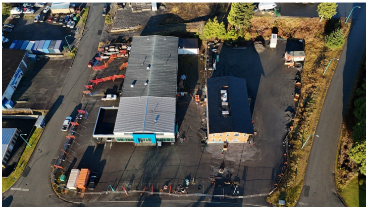
(Pictured above) The refurbished dealership building is now occupied by the City's Engineering staff, with occupancy of the fully new building anticipated over Summer 2026
