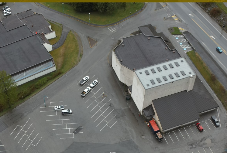
Repainting of the parking stall lines at the Lester Centre was one of many road painting projects completed around the City in 2025
