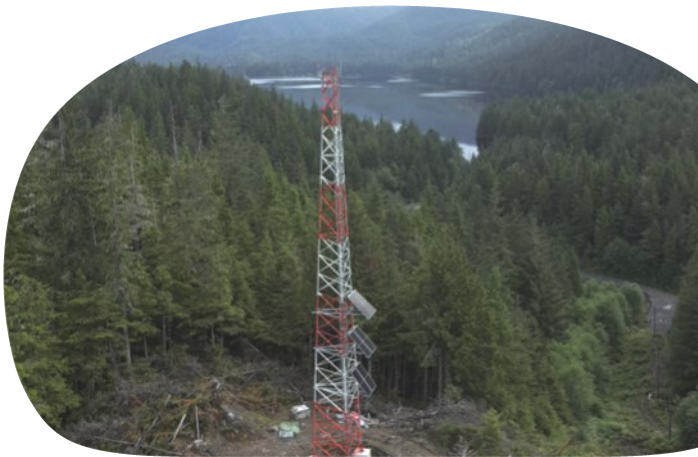
Pictured above —A new Supervisory Control and Data Acquisition (SCADA) tower has been installed to support enhanced communication to our water supply and treatment system
