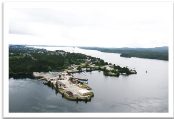
(Pictured Above: The City's distribution system runs beneath the harbour to Kaien Island)
