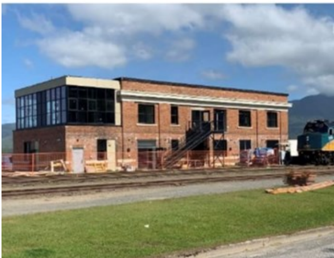
Refurbishment of the heritage rail building is now almost complete
