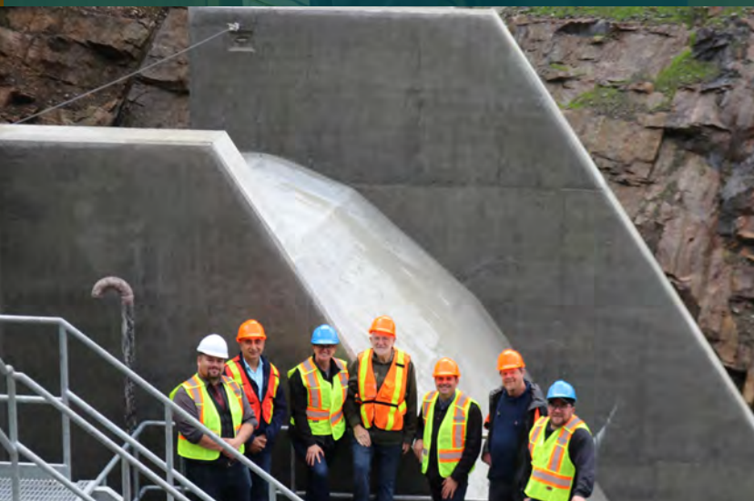
A long time coming—the City saw the structure of the dam replaced in the fall, and began drawing from our primary supply at Woodward lake early in 2023
