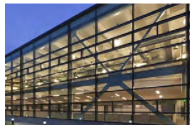
Visible structural elements
