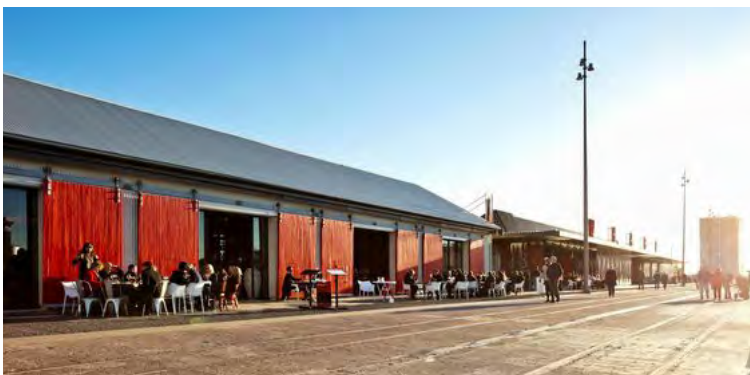
Frequent windows and entrances with industrial details.
