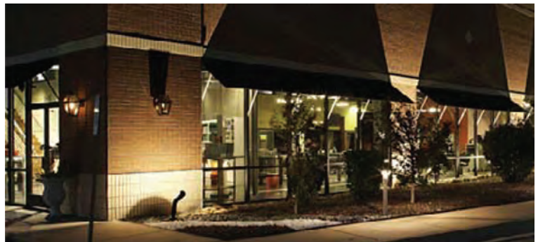
A combination of wall mounted lights, valence and surface lighting animate this building facade and adjacent pedestrian areas.
