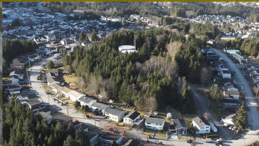
Full replacement of both water and sewer infrastructure occurred on the back half of Crestview Drive over 2025 as well as repaving of a first layer of pavement. Full repaving is occurring in 2026 of all of Crestview.
