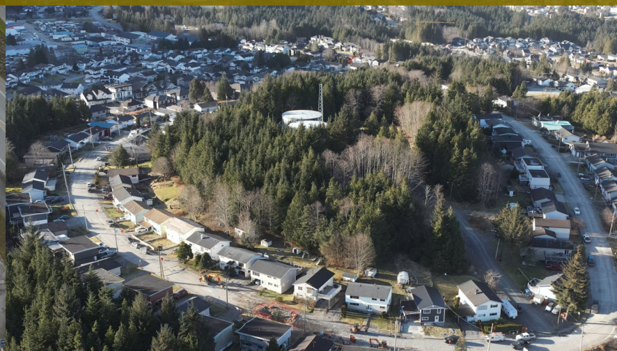
Full replacement of both water and sewer infrastructure occurred on the back half of Crestview Drive over 2025 as well as repaving of a first layer of pavement. Full repaving is occurring in 2026 of all of Crestview.
