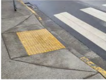
Letdown with a tactical walking surface indicator
