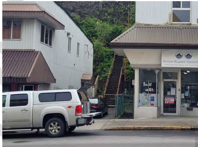
Closed staircase on 3 rd Avenue West
