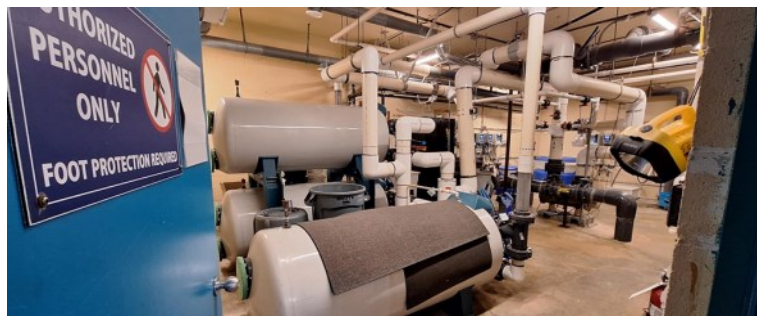
Pictured above: Filtration equipment at the Aquatic Centre
