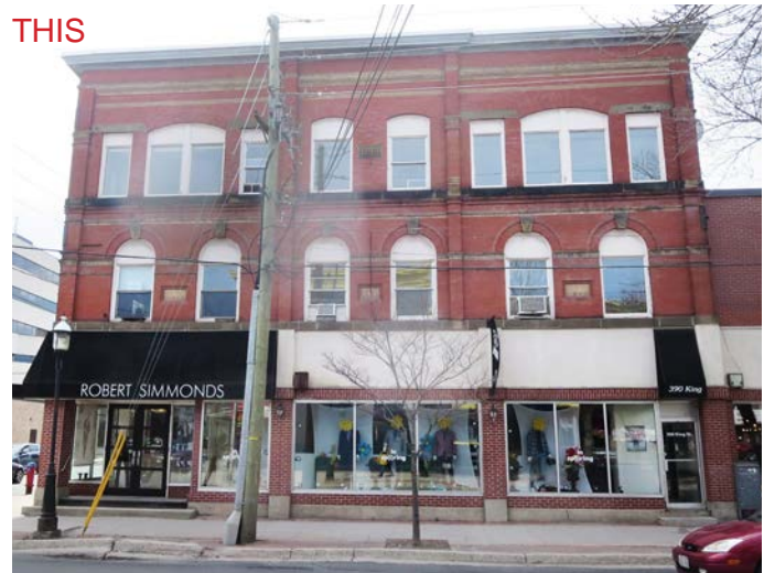
Many historic buildings are well articulated, having distinct zones in the facade (base-middle-top), strong horizontal and vertical datum lines (columns and cornices), and an emphasis on doors and windows.
