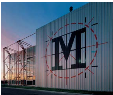
Vertical siding, exposed structure, distinctive sign and substantial full-height glass.
