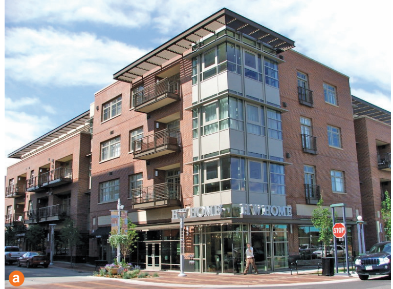
Building entrance is prominent in the facade through techniques including modest increase to street wall height, change in materials and fenestration at corner, roof line overhang element, ground level canopy providing weather protection, and corner access.
