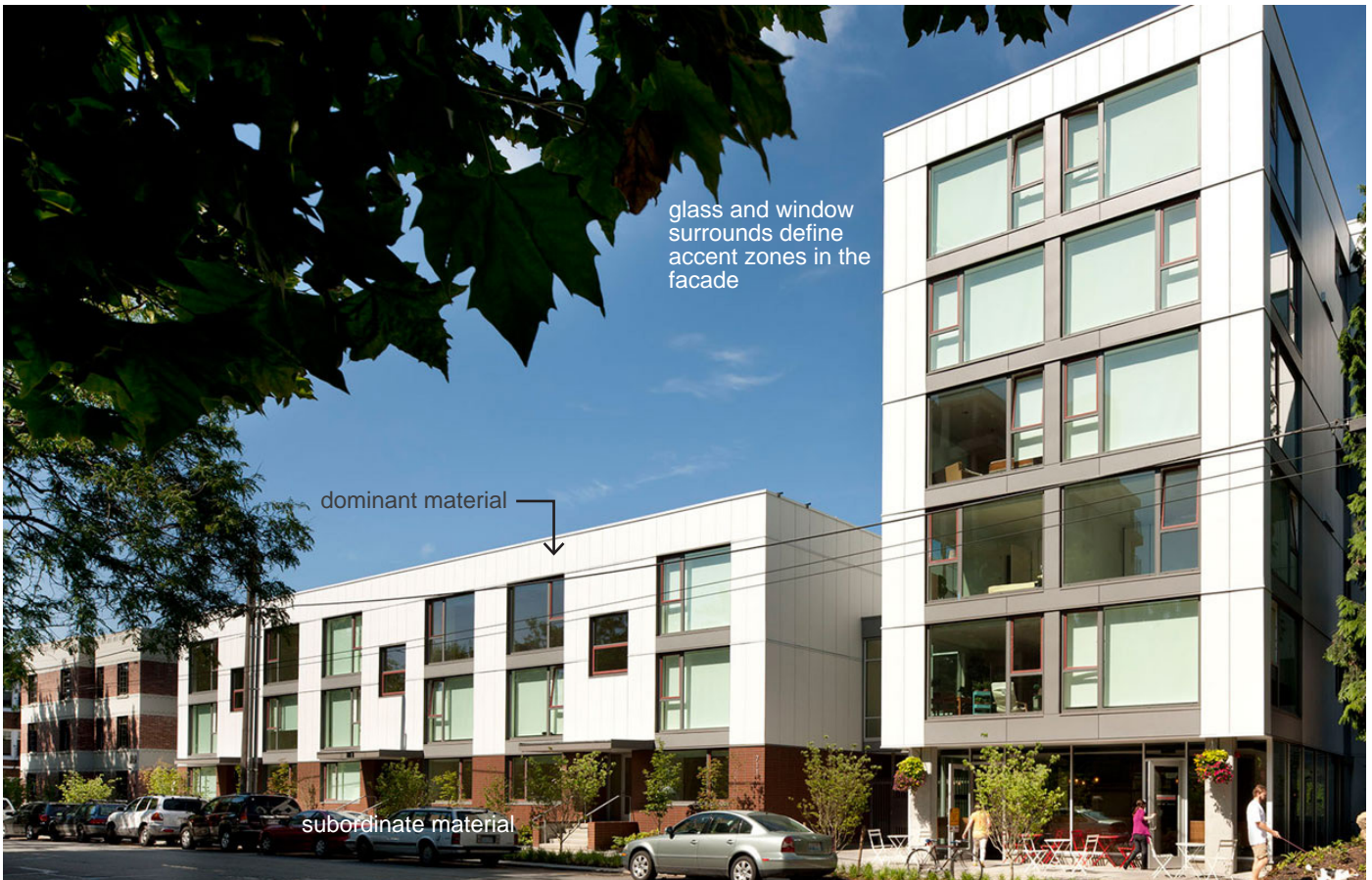
The interplay of materials helps to activate this facade and act as datum lines defining zones.
