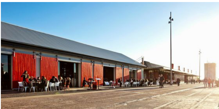
Frequent windows and entrances with industrial details.
