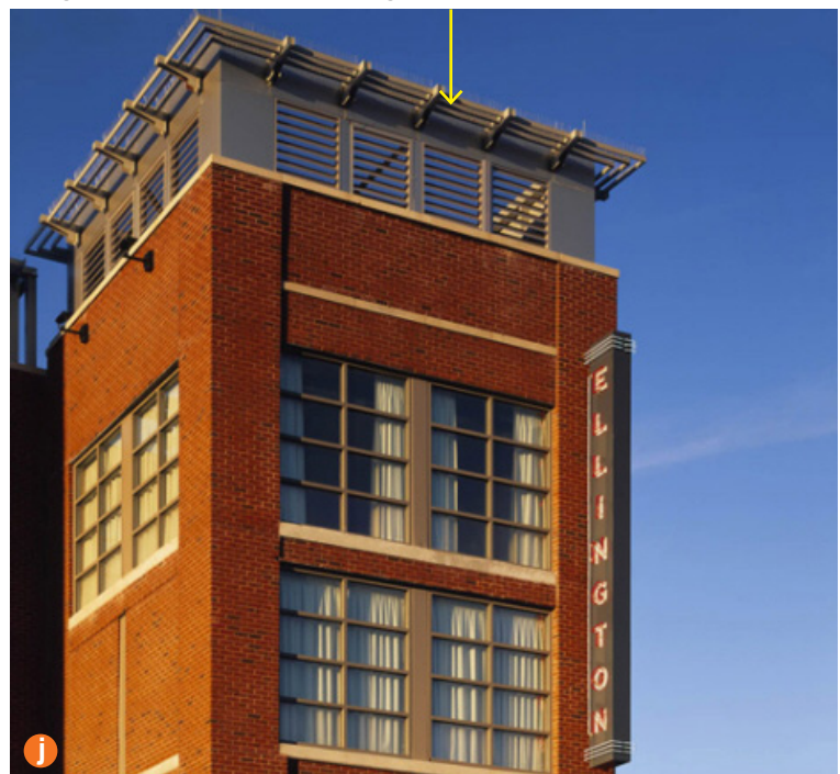
Screening of mechanical equipment is integrated with the building design and is part of the building's top.
