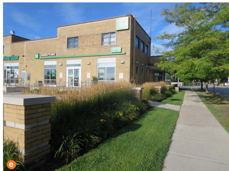
Surface parking adjacent to the sidewalk screened by hard and soft landscape.
