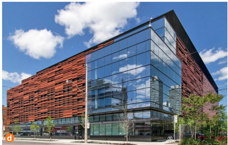
Public art treatment for upper level facades of a data centre.
