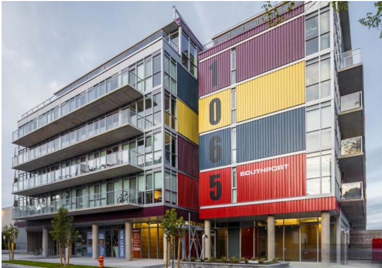
Corrugated metal is used creatively as a reference to shipping containers. It is crisply detailed, and transitions neatly to other materials such as glass.
