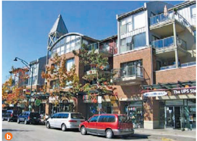
Vertical and horizontal articulation, through changes in plane, reduce the perceived scale of large buildings.
