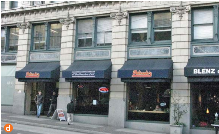
Sensitive incorporation of new weather protection minimizes obscuring of the building facade and historic detailing.
