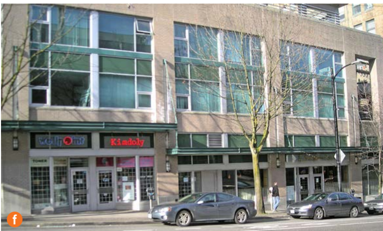
Weather protection organized in modules and terraced to step down a slope.
