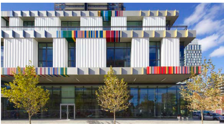
Public art can be integrated with the building's structure and expression (above), or be stand-alone (top).
